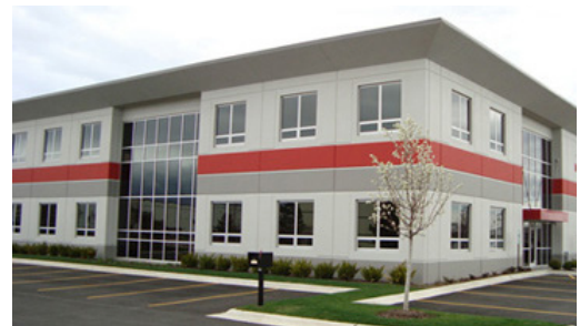
An example of a high quality office building using variations in building color, projections and windows to break up long walls.
