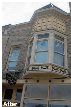
Before After Original brick facades should not be covered by siding. Above, before and after images show a restoration project that revealed the original brick and architectural details
