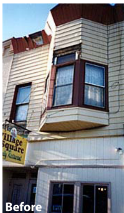
Before After Original brick facades should not be covered by siding. Above, before and after images show a restoration project that revealed the original brick and architectural details
